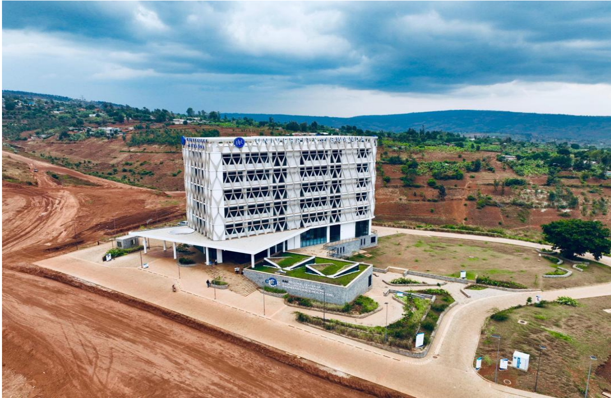
FIGURE 6.0: EXISTING BUILDING AND ITS VICINITY
