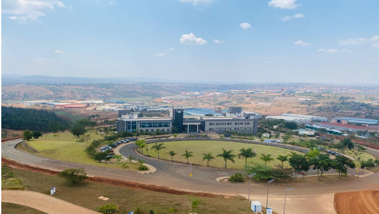
FIGURE 7.0: ROUNDABOUT AT THE PROJECT AREA
